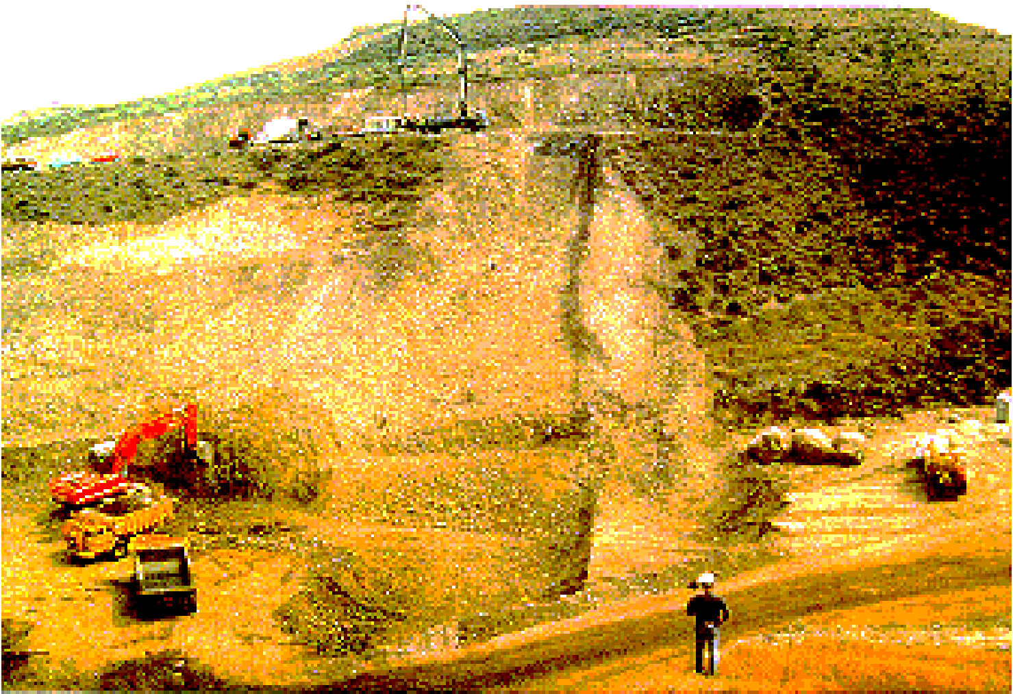
Photo C-1. Excavating basalt rock foundation
