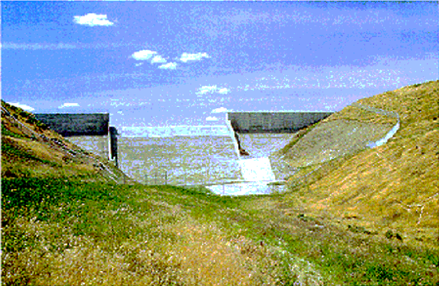
Photo C-7. View of the completed Zintal canyon dam
