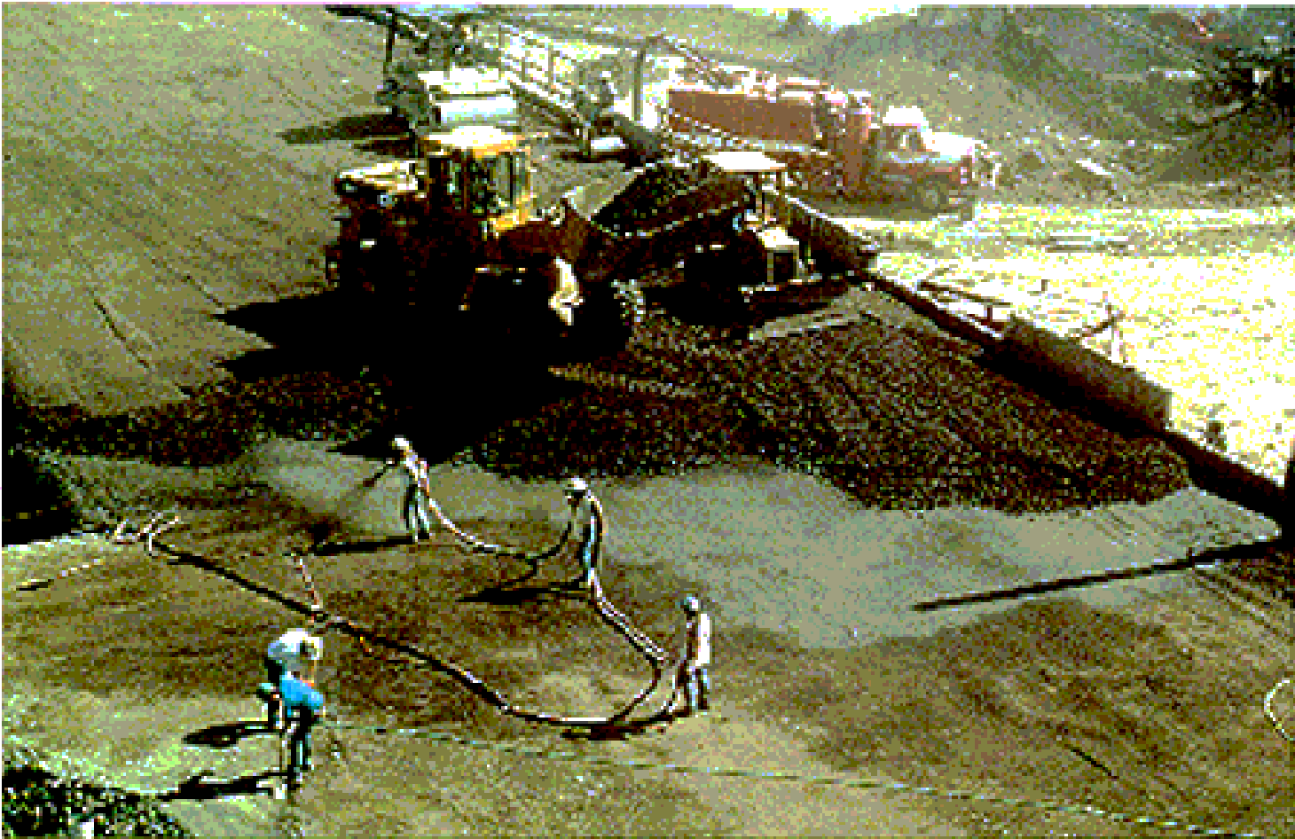
Photo C-5. Typical RCC placement process of loader transport
