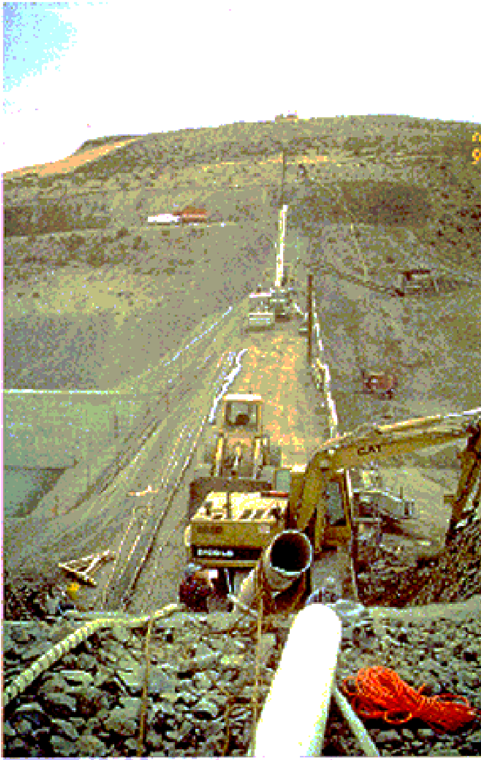
Photo C-6. Constricted placement conditions for RCC placement
