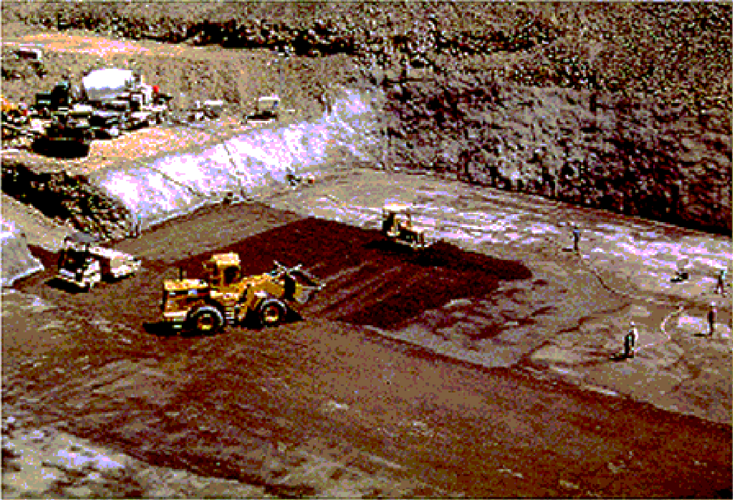
Photo C-3. Transportation, spreading, and compacting RCC
