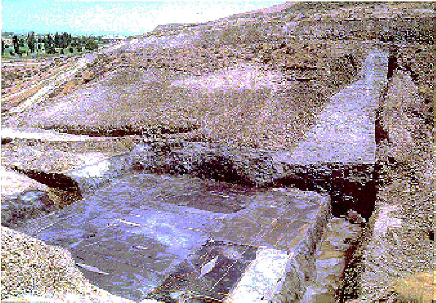
Photo C-2. Foundation after placement of concrete and shotcrete
